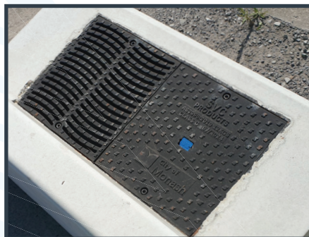
▲ Two-part insert featuring Class C pedestrian-safe grate and solid cover
