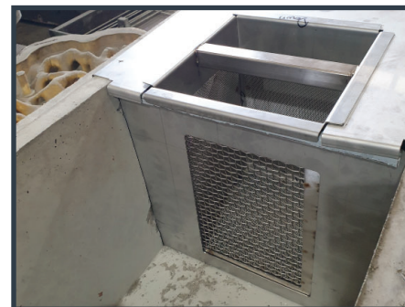
▲ Easily removable steel silt basket with 6mm mesh screen at front plate
