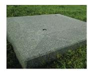
Custom blasted finish for the City of Yarra, featuring a charcoal base colour with an exposed white stone aggregate.
