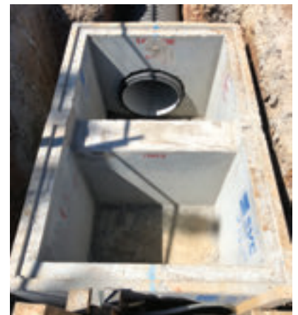
Before and after: On-site adjustments to two stock pits results in the creation of a dual chamber overflow system.
