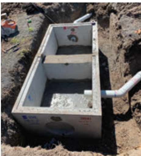
Image: Melbourne Plumbing & Gasfitting
