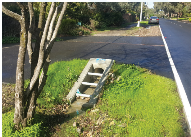
Driveable endwalls installed alongside a road in Upper Plenty.
