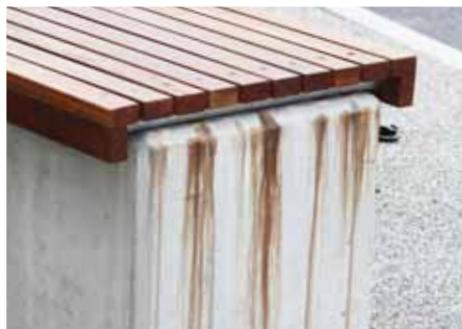
Untreated timber can often cause unsightly tannin stains on the concrete components beneath.
