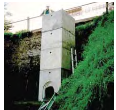
Multiple pit risers stacked to extend the height of a standard pit
