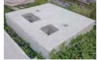
Electrical transformer support base
