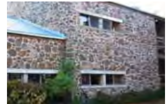
Precast concrete building lintels installed in Kyneton
