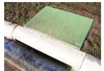
Side entry GridLite frame and cover set in situ behind kerb lintel
